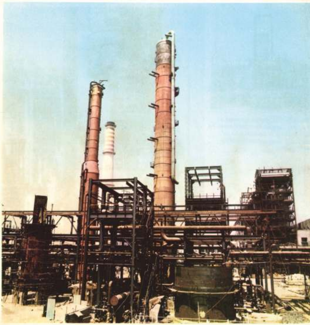
The various stages of site assembly of shop fabricated Benfield Regenerator and Benfield Absorber
