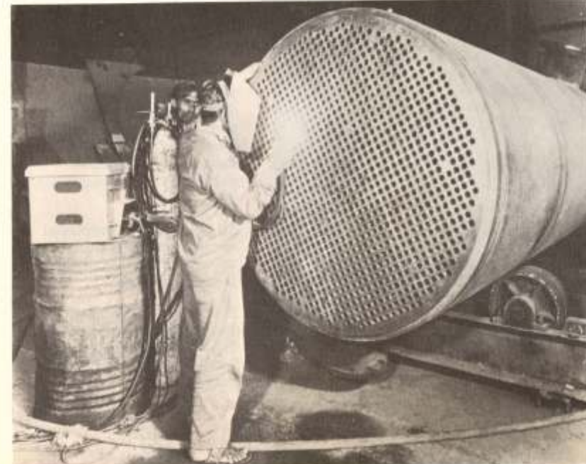
Stainless steel ammonia condenser under fabrication for heavy water project
