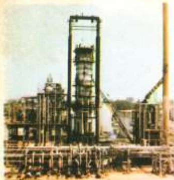
The various stages of extension of height to Vacuum Pipe Still Column T-1 at a Refinery in Bombay with an especially designed derrick pulley arrangement
