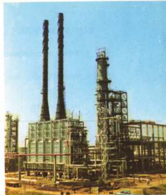
Crude heater constructed for 3.5 million tonne Petroleum Refinery in Gujarat
