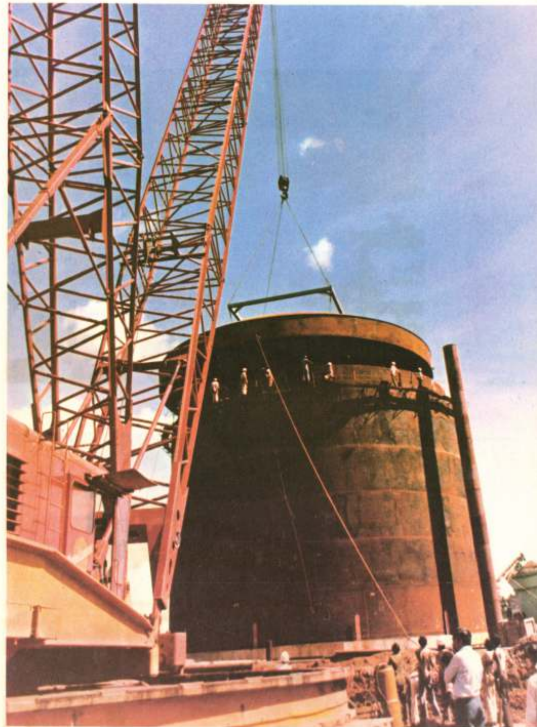
3,000 metric tonne double integrity ammonia storage tank under final assembly at State Fertilizer Mfg. Corp. Sri Lanka.
