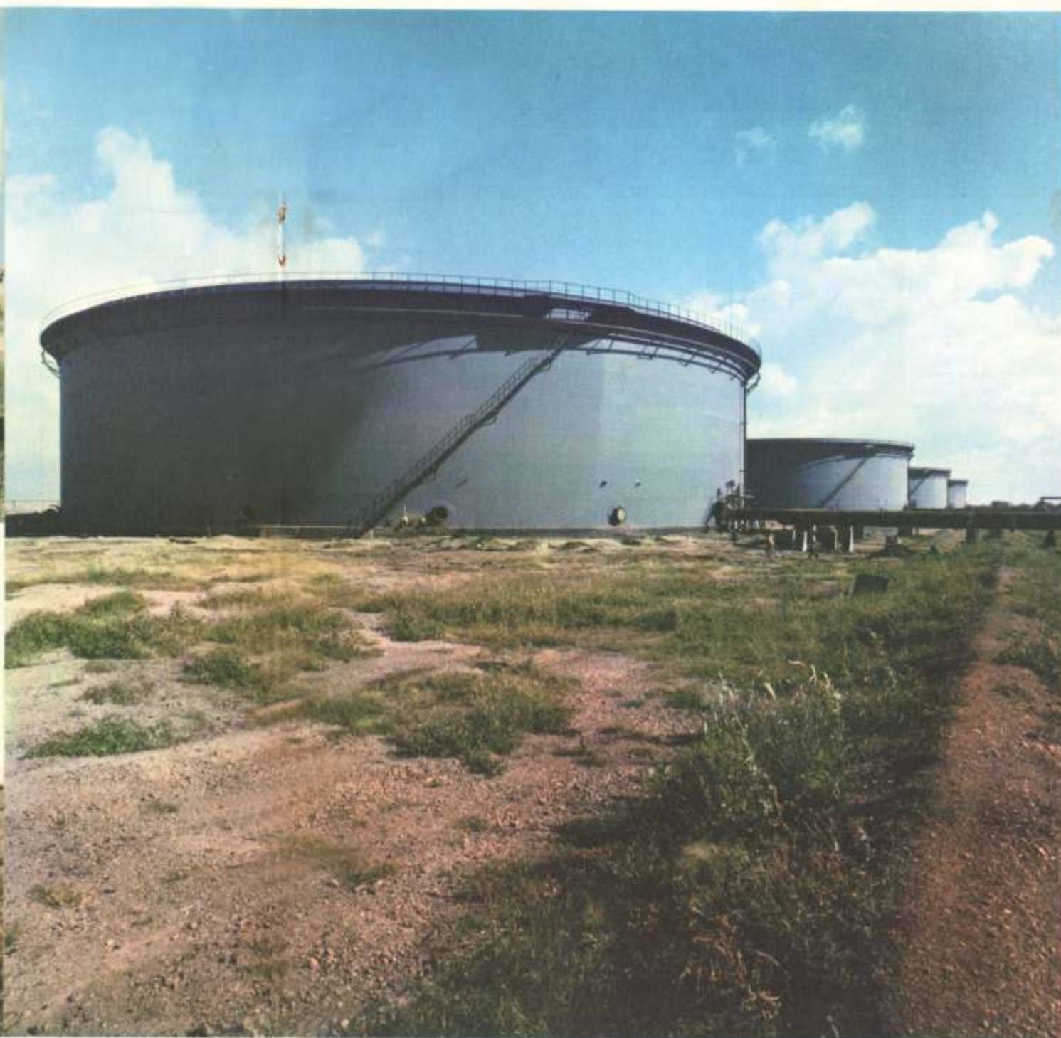
Crude Oil Storage Terminal at Vadinar where 8 x 90,000 M 3 tanks were constructed
