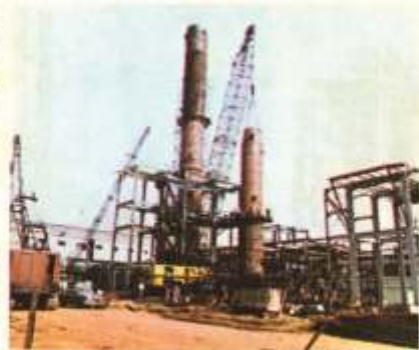
The various stages of site assembly of shop fabricated Benfield Regenerator and Benfield Absorber
