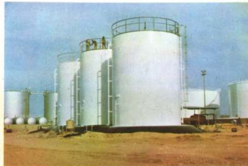
A view of 3 nos. 400 M 3 Fire Water tanks For KAFCO, at Kuwait Airport.
