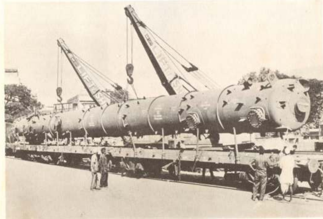
A 1.8 M dia x 39 M long shop-built fractionating column being shipped to a Fertilizer Project site
