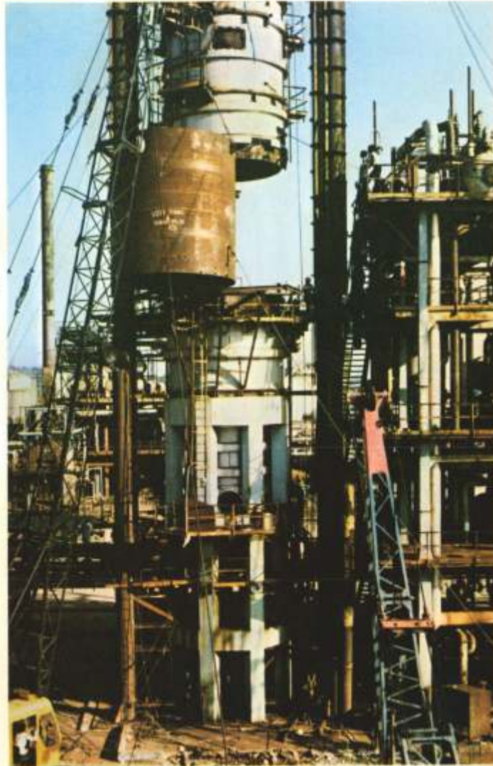
The various stages of extension of height to Vacuum Pipe Still Column T-1 at a Refinery in Bombay with an especially designed derrick pulley arrangement
