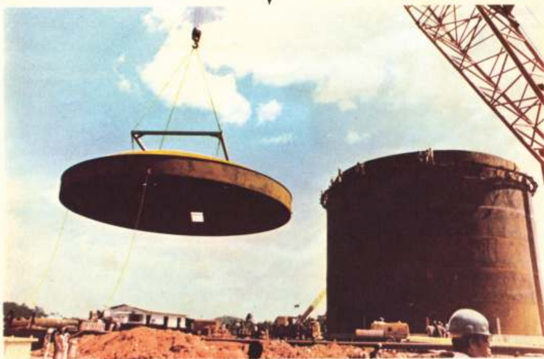
3,000 metric tonne double integrity ammonia storage tank under final assembly at State Fertilizer Mfg. Corp. Sri Lanka.
