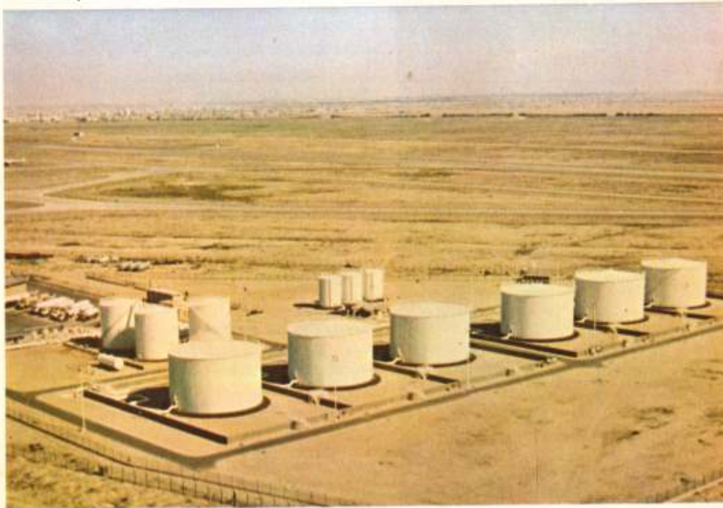
A view of aviation fuelling depot constructed on a turnkey for KAFCO, Kuwait
