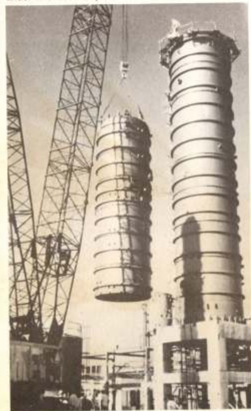
A 4.75 M dia x 40 M high fractionating column— under final assembly at a Petrochemical Complex
