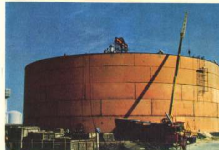
A view of 3 nos. 400 M 3 Fire Water tanks For KAFCO, at Kuwait Airport.
